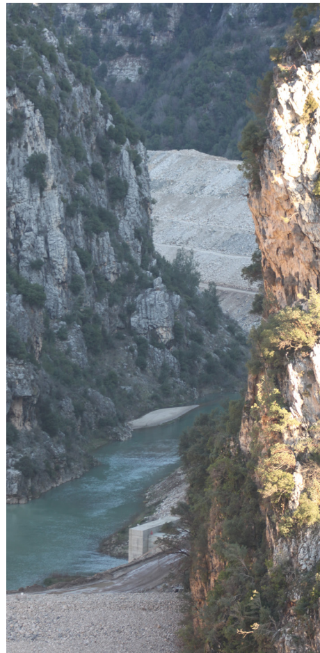
Janneh Dam under construction. Photograph: by author
